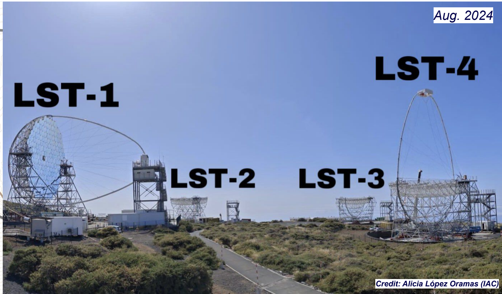
CTAO-North already under construction
