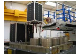
A single TKR Module being lowered onto the Grid, next to two TKRs that have already been installed. Empty Grid bays are filled with mass dummies.
